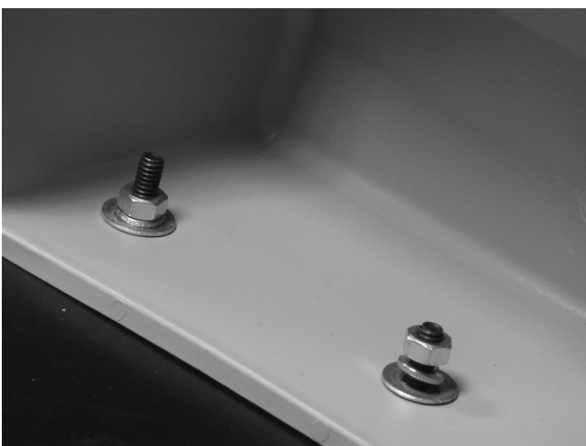
Figure 19a - Plastic Bucket Installation
